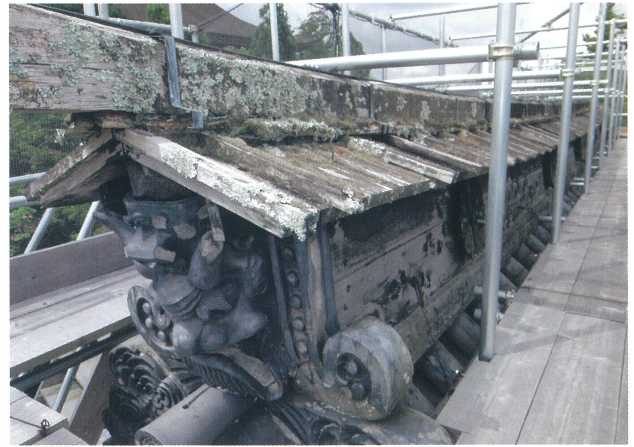
箱棟の腐朽
