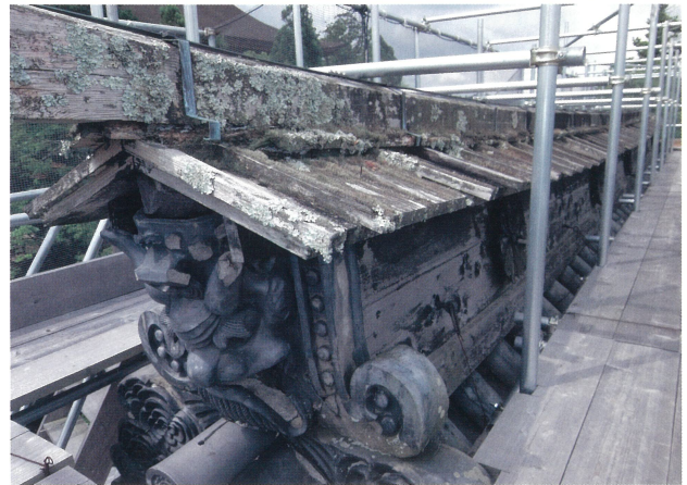
箱棟の腐朽
