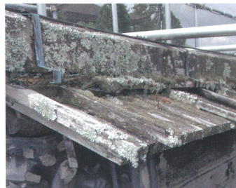
▲箱棟の腐朽
